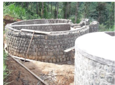
URF beside SSF tank
