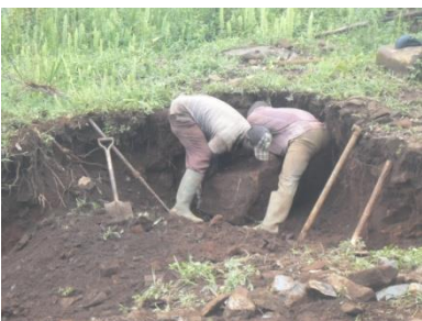
Extracting stone after earth excavation
