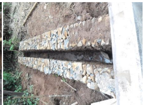
Intake dam wall
