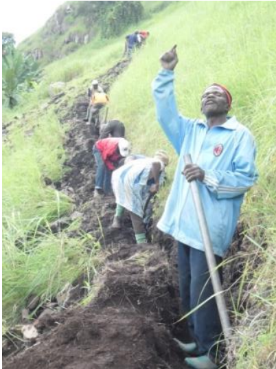
Community work-excavation of pipeline trenches through stony sections
